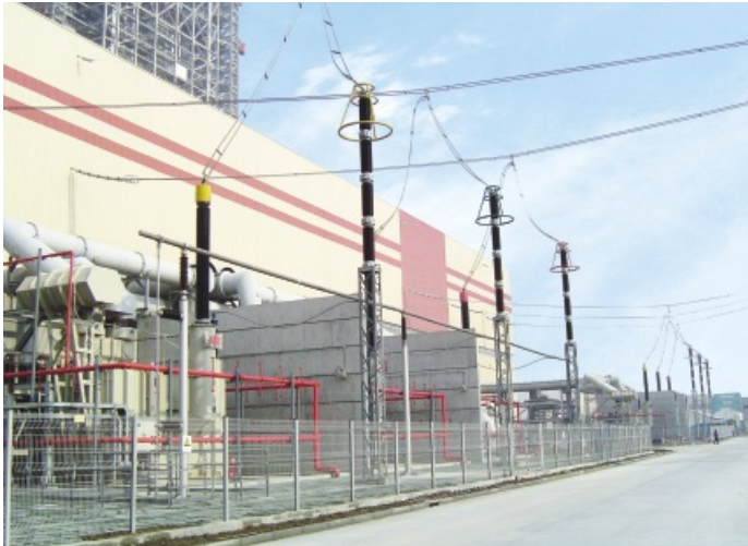
上海外高桥电厂 Shanghai Waigaoqiao power plant
