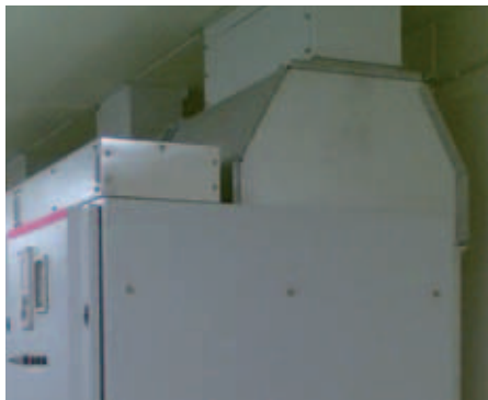
Figure 59: Example of switchgear with gas duct with outlet (total height of the switch-gear is 2675 mm for 12-17,5 kV up to 40 kA)
