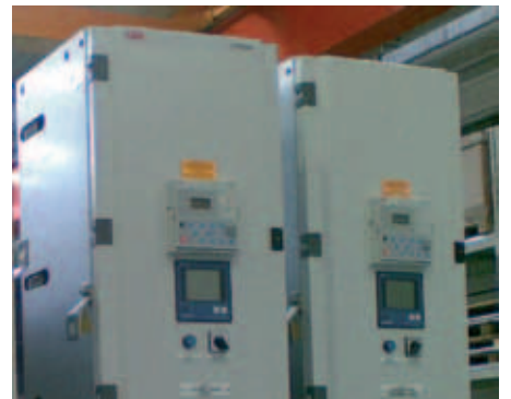
Figure 60: Example of UniGear ZS1 with higher LV compartment (1100 mm)
