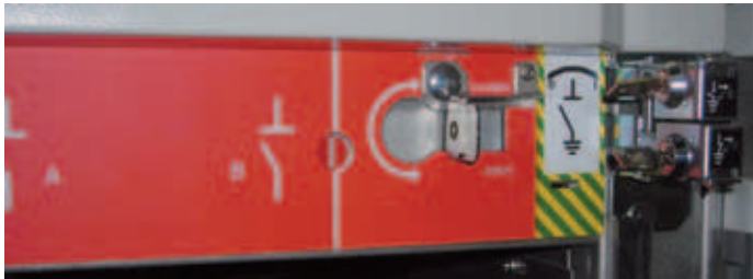
Figure 65: Front panel with operating slots of busbar-disconnector
