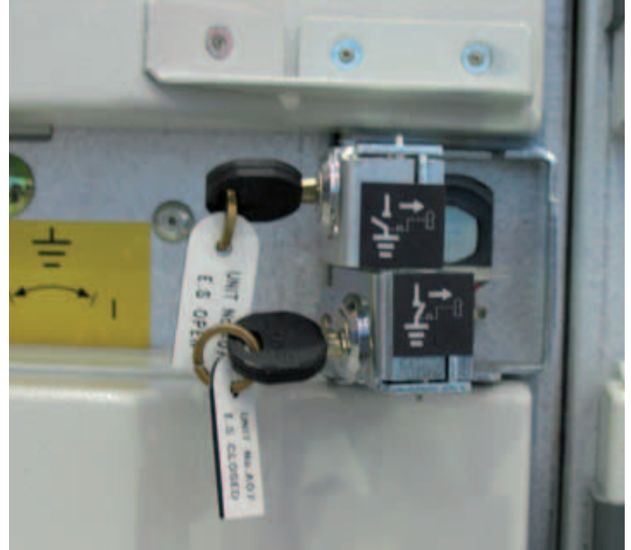
Figure 6: Double key lock on earthing switch
